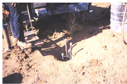
Installation of a Three Tier Probe
