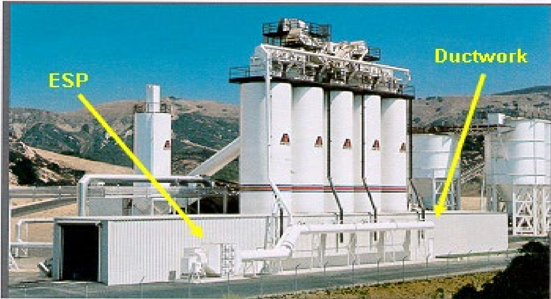
DUCTWORK TO ELECTROSTATIC PRECIPITATOR
