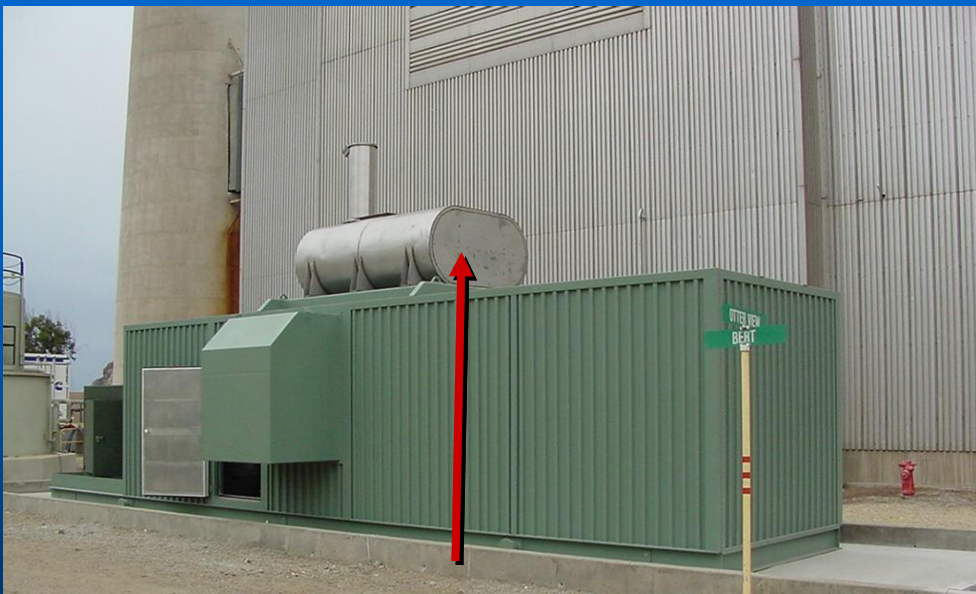
Diesel Particulate Filter (DPF)
